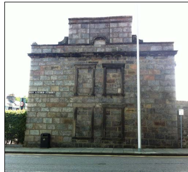
Example of blocked up windows in Ferryhill
